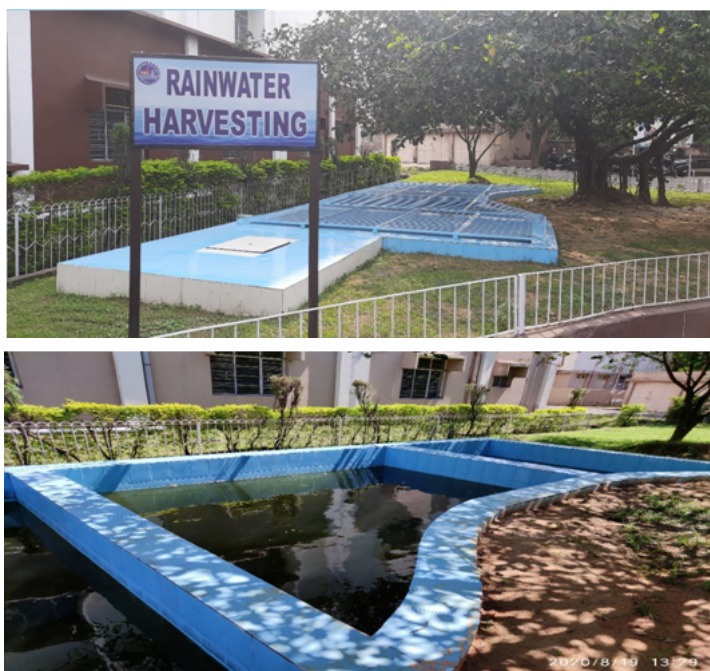
Fig. 9.11c: Rainwater harvesting system.
